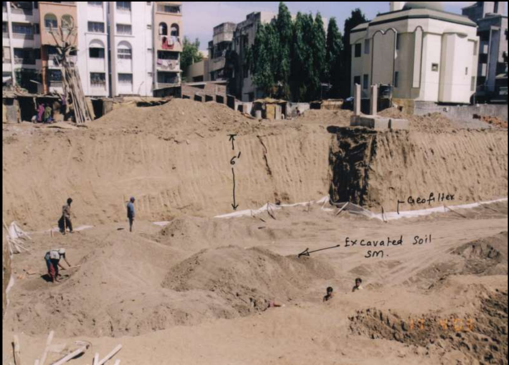
Spreading Layer of Same Soil to be Compacted over Filter.
