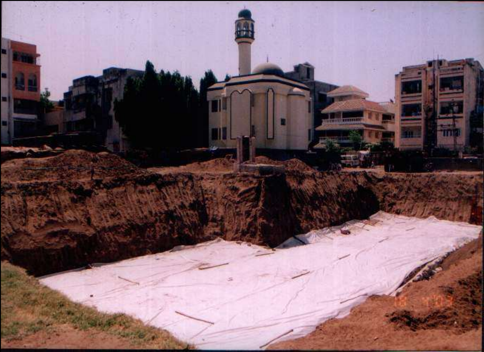
Providing Geofilter for Separation or as Reinforcement
