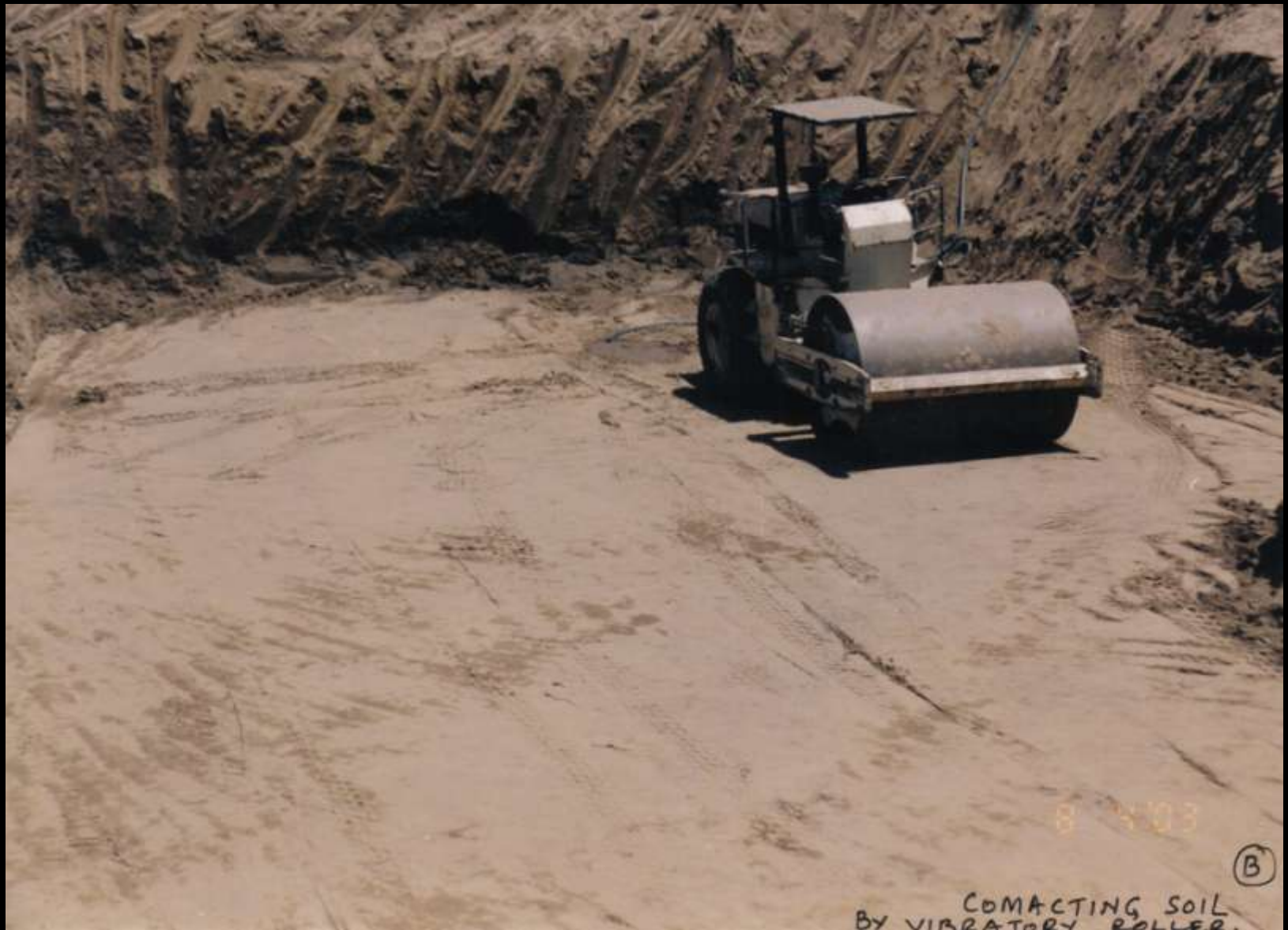
Compaction of Bottom of Excavation by 10 T Vibratory Roller
